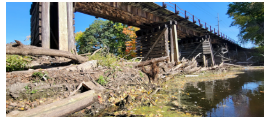
Grand River Railroad Bridge Engagement North Lansing, November, 2022
